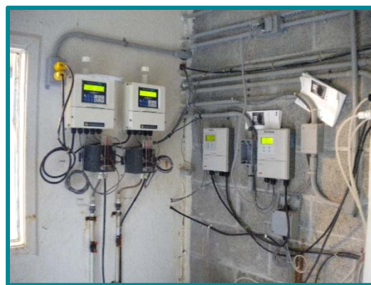
Figure No.2: Chlorine Injection at the Royston Chlorination Station.
