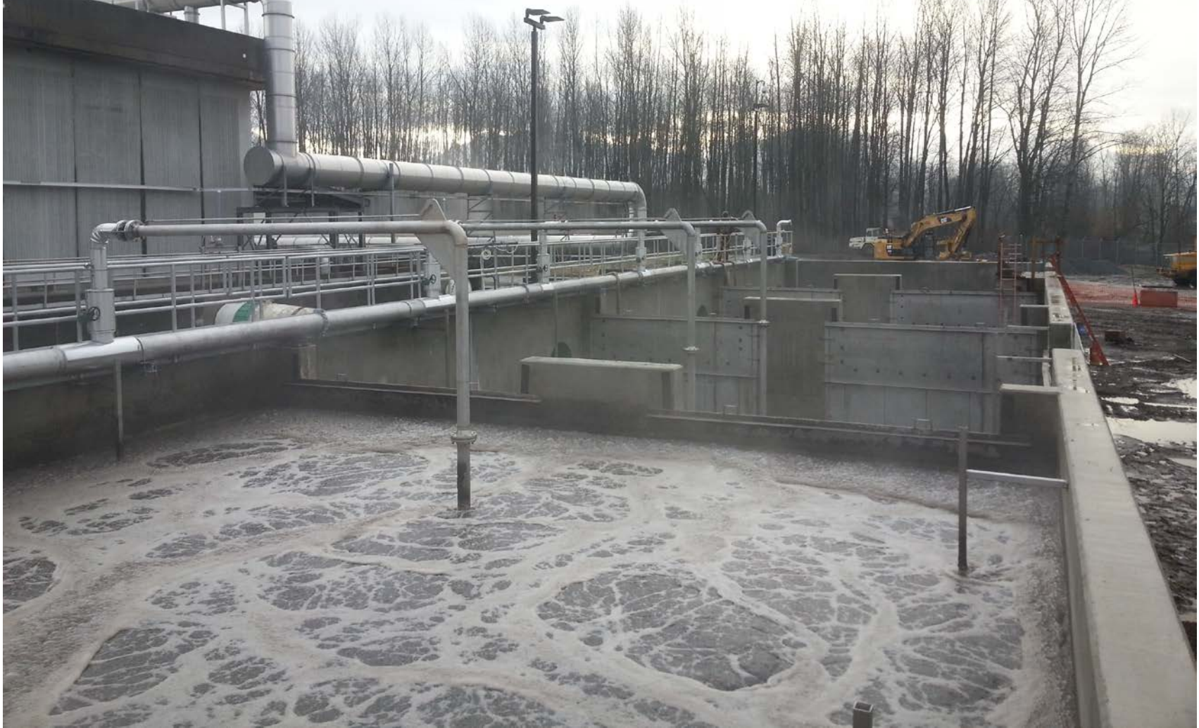
Activated Sludge Aeration Basins
