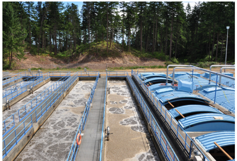
The bioreactors (left) will have covers installed, like those blue lids already in place over the primary clarifiers (to right).
