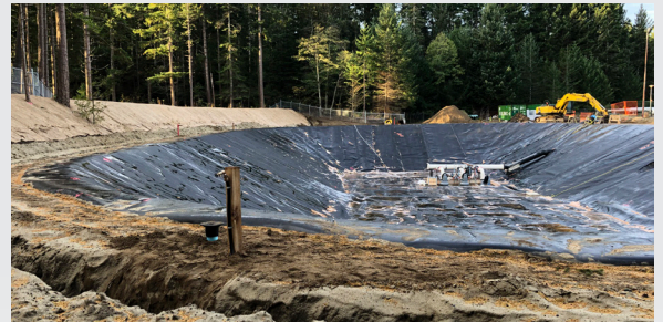
Installation of new EQ basin is nearing completion.
