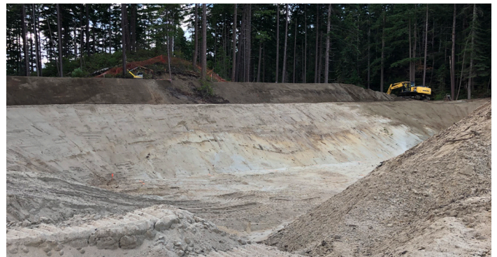
Construction moving ahead on the new EQ basin and berm.
