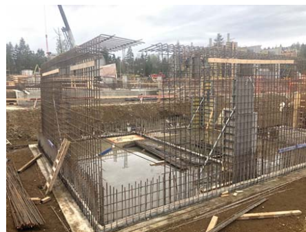
Left to Right: Raw Water Transmission Main, Water Treatment Plant Underground Facilities, Water Treatment Plant Clearwell Foundations
