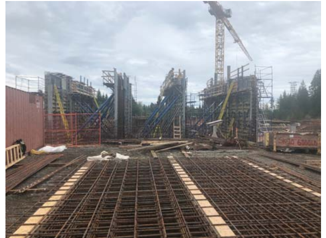
Water Treatment Plant: Flocculation Basin Wall
