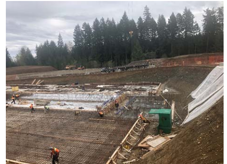
Left to Right: Raw Water Transmission Main, Water Treatment Plant Underground Facilities, Water Treatment Plant Clearwell Foundations
