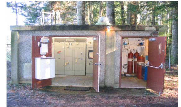
Current water treatment building
