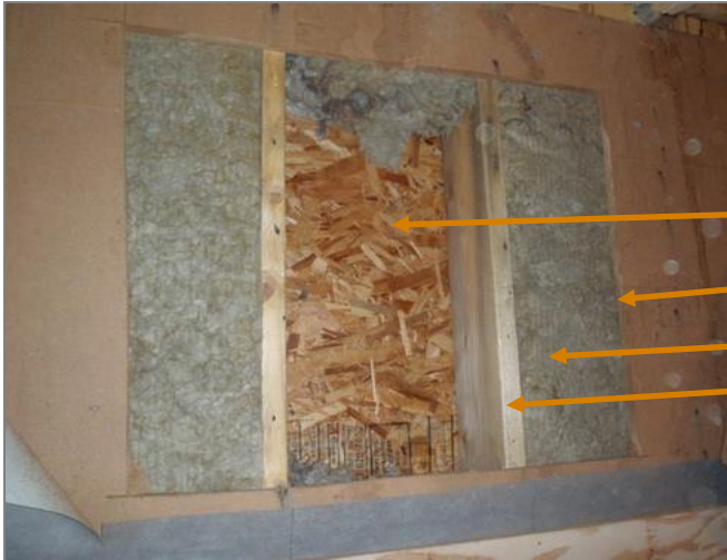
Figure 2.13 Opening 4 bottom of wall GL 1/D Moisture Content Readings 10% MC OSB interior sheathing 20% MC back side of Agepan dry insulation 17% MC outboard face of stud
