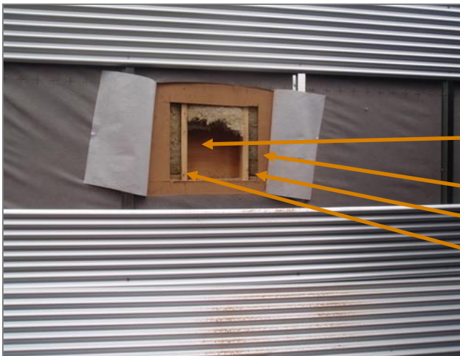
Figure 2.12 Opening 3 bottom of wall GL 1/G Moisture Content Readings 10% MC plywood interior sheathing 20% MC back side of Agepan dry insulation 17% MC outboard face of stud
