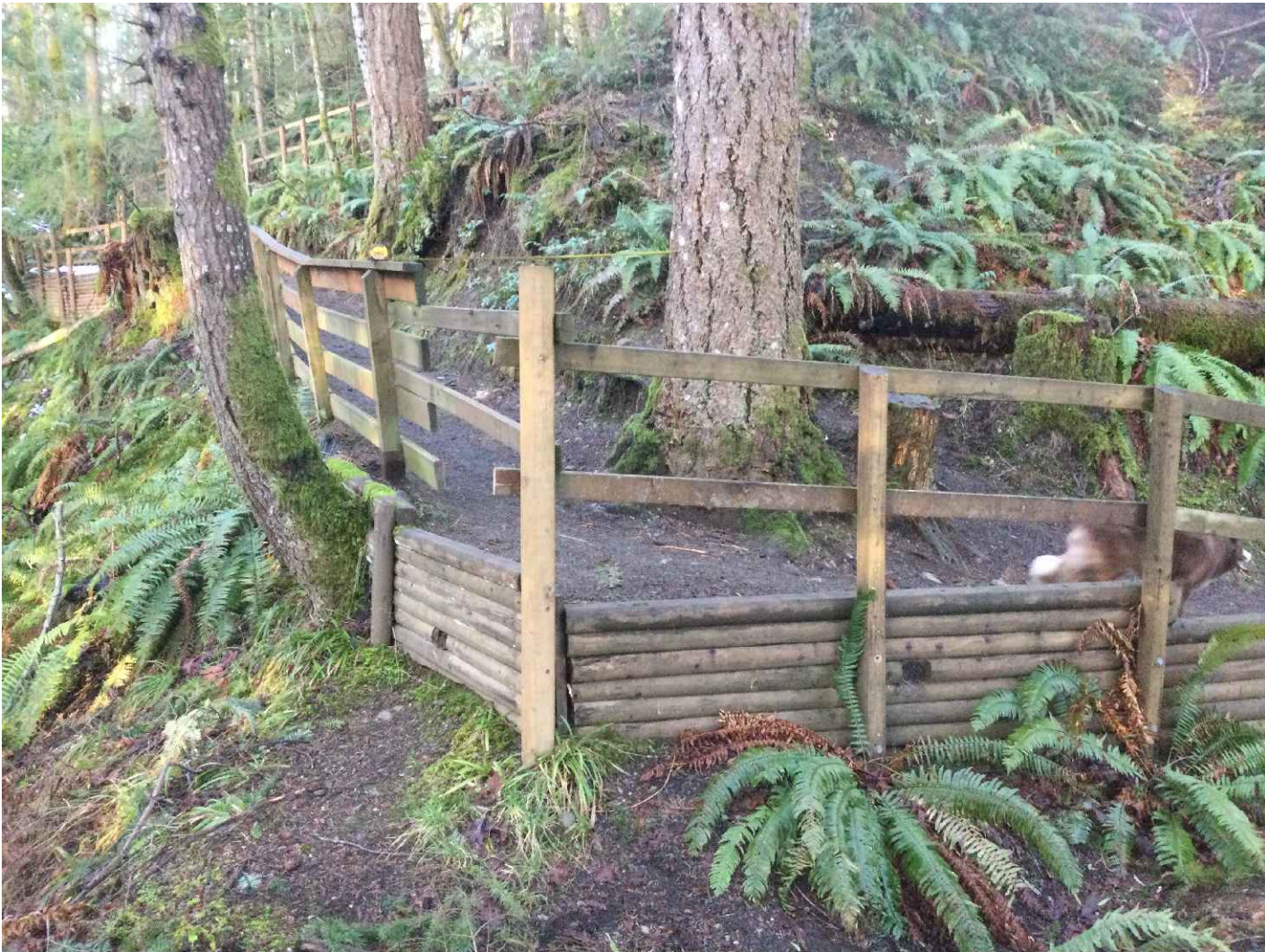
PHOTO #2 APPROXMIATE STA 0+095
