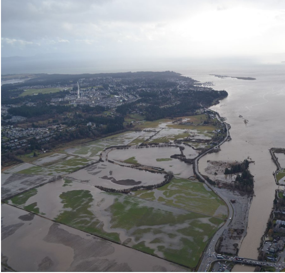
Figure 2-2: Flooding of the project area, seen from the air, on 9 December 2014. Source: City of Courtenay.
