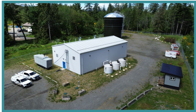
Union Bay Water Treatment Plant
