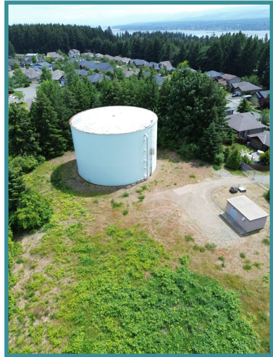
Comox Reservoir and valve house.
