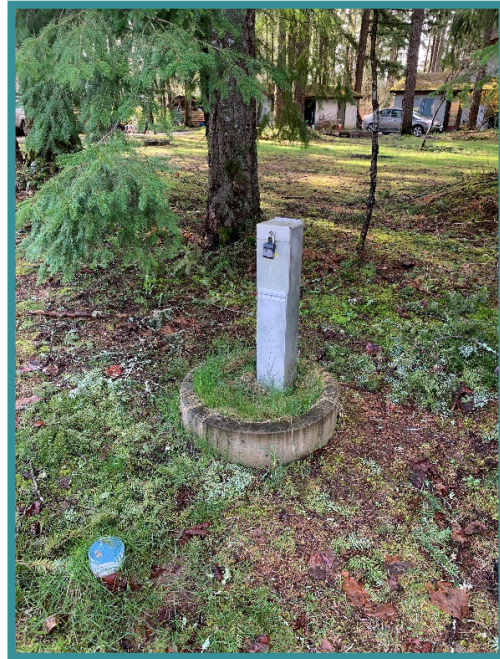
A sample station in the distribution system.
