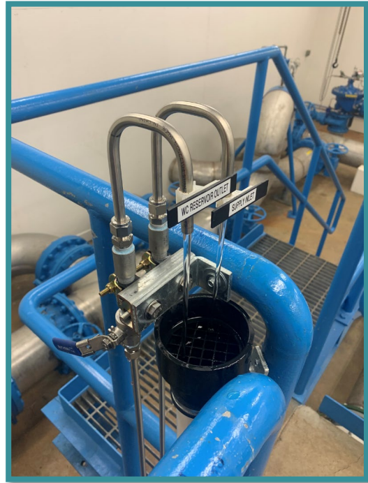
Sample taps at West Courtenay Reservoir.
