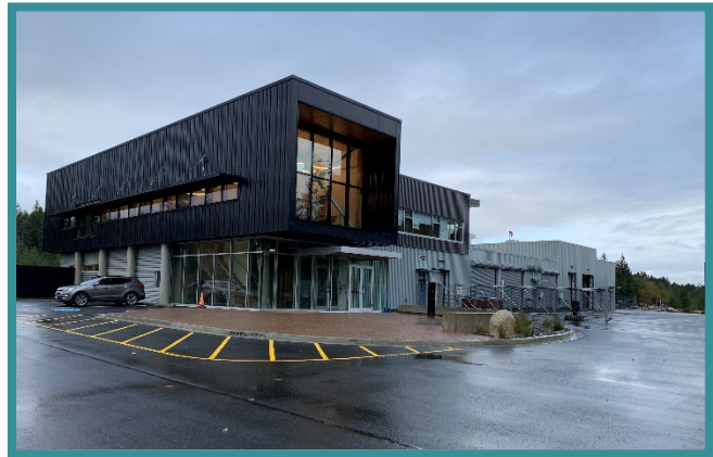
Comox Valley Water Treatment Plant
