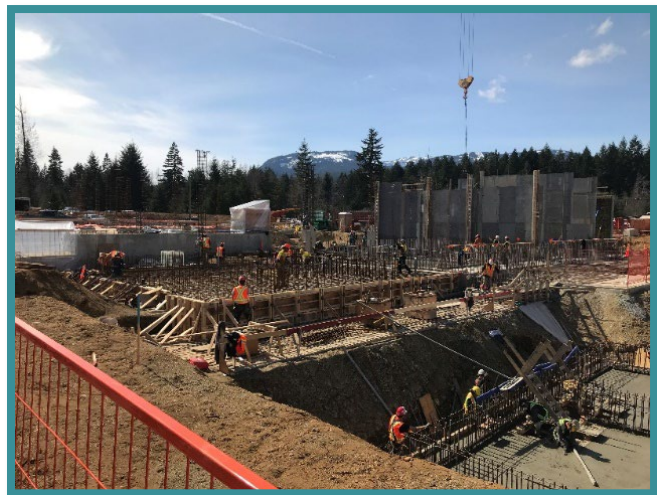
Construction of the water treatment plant in 2020.
