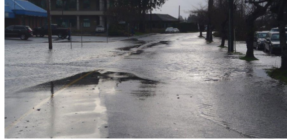
Figure 2-3: Flooding of Comox Road near 5th St, on 9 December 2014. Source: City of Courtenay.
