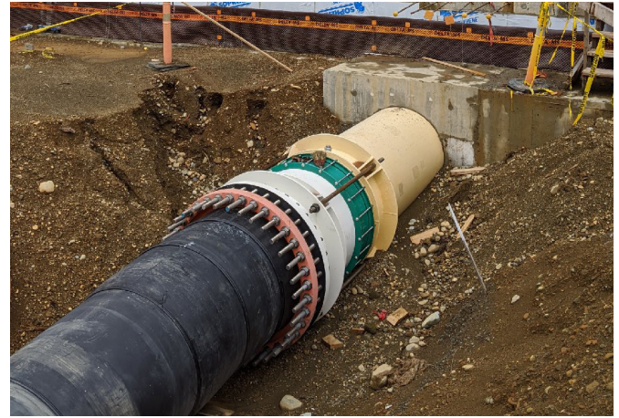
Raw water transmission main connection to the water treatment plant
