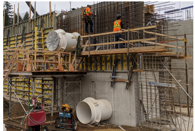
Clearwell discharge/joint that will connect to the treated water transmission main
