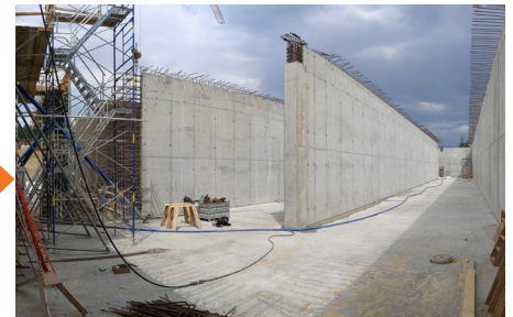
Concrete is poured and walls are installed at the clearwell. (Jul. 2020)
