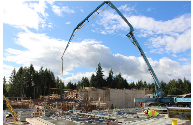
Crews pouring concrete for the filter chamber at the Water Treatment Plant
