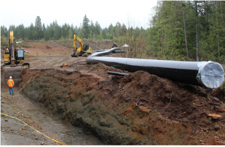
Installation of the raw water transmission main started earlier this year. (Apr. 2020)
