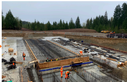
Clearwell structure starting to take shape. (Apr. 2020)
