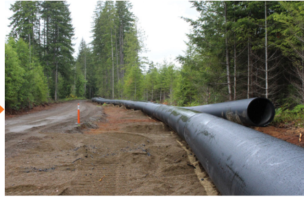
This transmission main will move water from the raw water pump station site at Comox Lake to the new treatment plant. (May 2020)
