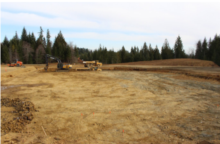
Excavation of the clearwell – a large reservoir which feeds the pipeline that connects to the existing distribution system. (Mar. 2020)
