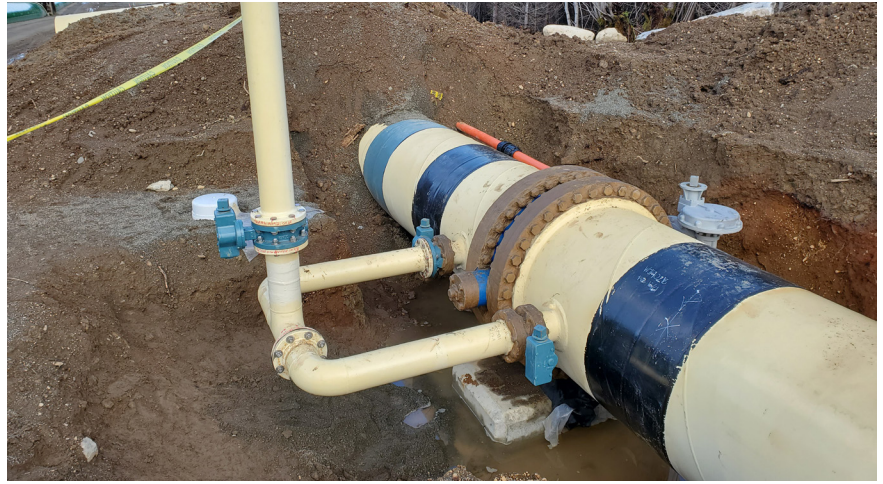
March 2021: One of three isolation valves along the length of the treated water transmission main.
