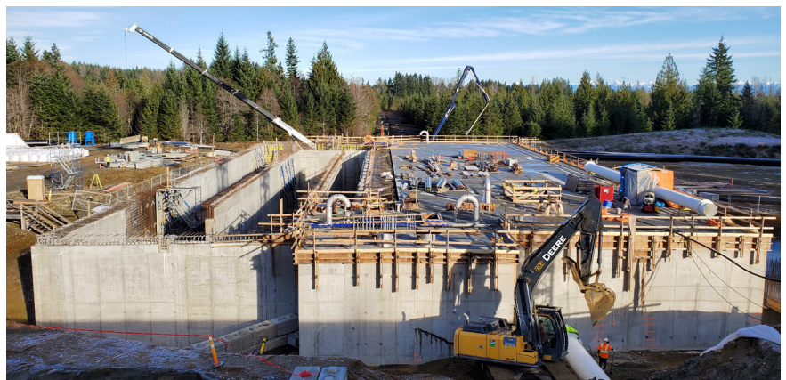
December 2020: A birdseye view of the clearwell with Cell 1 complete, and before completion of Cell 2. Inside the clearwell are the internal baffles, which provide a long travel path and contact time for the water after chlorine disinfection, ensuring it is safe to drink.
