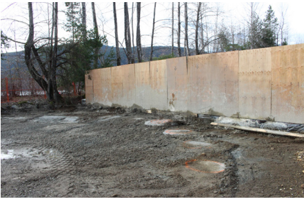
49 piles were drilled down into bedrock to make up the pump station wet well/tunnelling shaft. (Feb. 2020)
