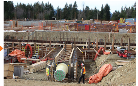
The pipe that will move treated water into the clearwell, a large reservoir which feeds the pipeline to connect to the existing distribution system. (Mar. 2020)
