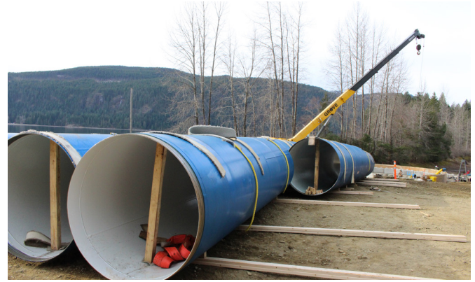
Pipe has arrived on site, for the marine pipeline that will transport water from the intake in Comox Lake to the pump station. This pipe will be tunnelled into the lake.
