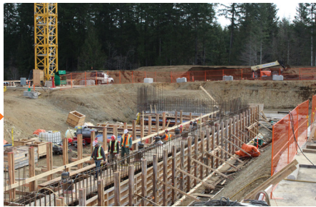
Crews are now working on wall installation for the new water treatment building. (Mar. 2020)
