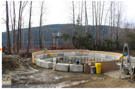
The piles were connected to create a solid outside wall for the wet well/tunnelling shaft. (Mar. 2020)
