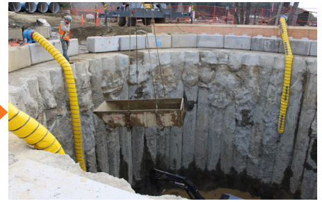
Excavation work is completed to the depth of the wet well/tunnelling shaft, approx. 12m. (Mar. 2020)
