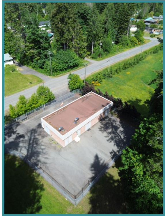
Black Creek/Oyster Bay Water Treatment Plant.
