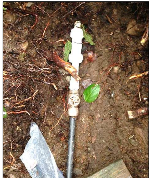
November 29, 2017 4356 East Road - Watermain side Unusual PVC service connection. PVC (thin walled) snapped when attempting to shut off curb stop. Installed compression fitting.
