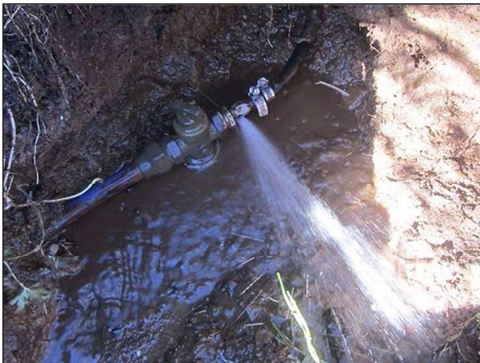
August 28, 2017 3941 East Road – Leak at curb stop, customer side.
