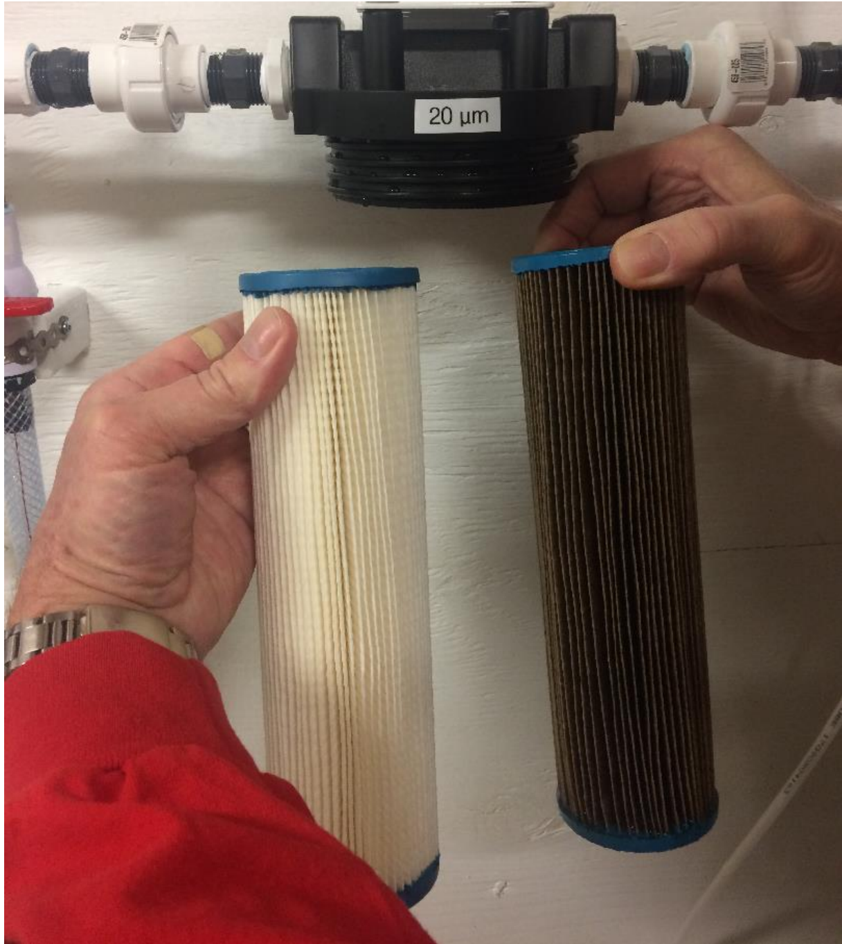
Figure 3: 20 Micron Cartridge (clean vs dirty)
