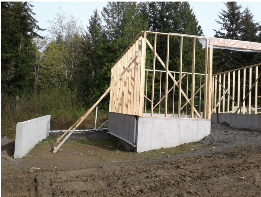
Figure 5: Accessory Building with Carport
