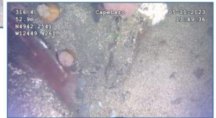
Photo 64 – North Wye Welded seam Leaking
