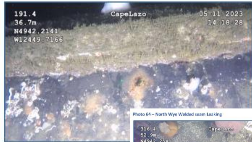
Photo 74 – Close Up of Possible Corrosion on Exposed Steel Pipe
