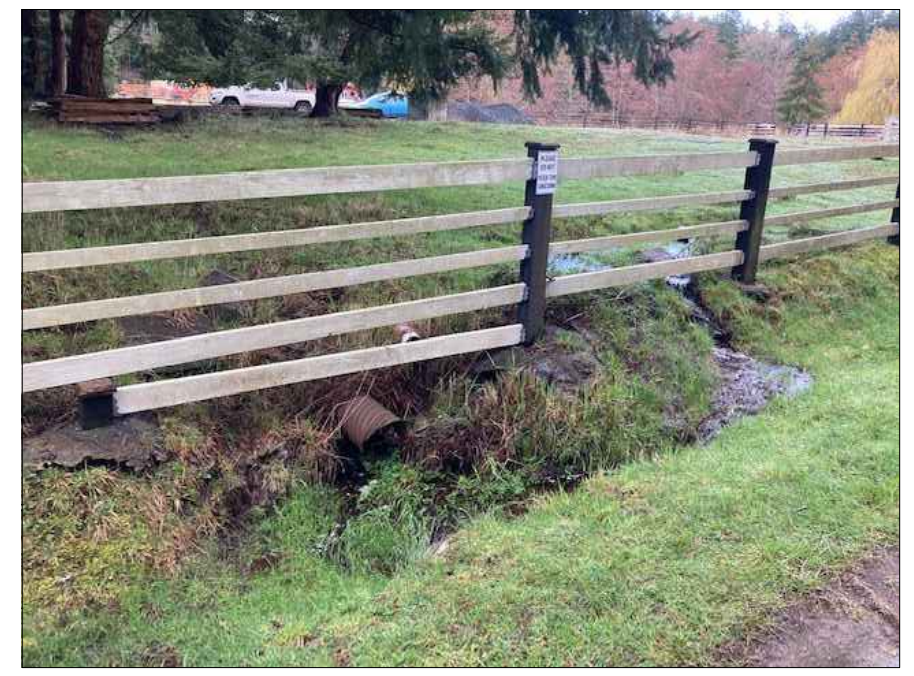
EXISTING DRAINAGE SUMP @ STA. 3+390
