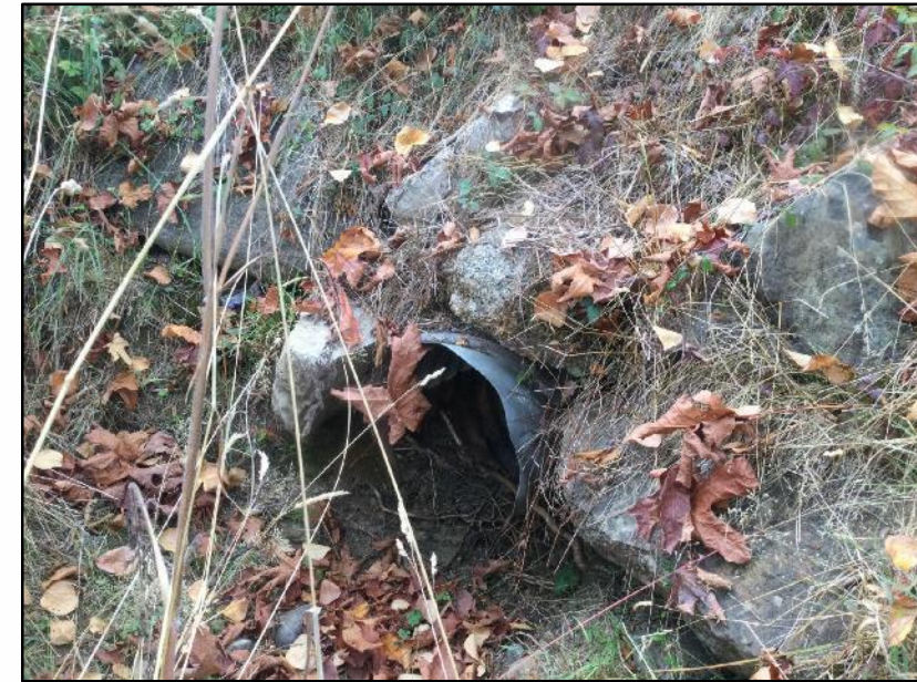
Unnamed ditch crossing
