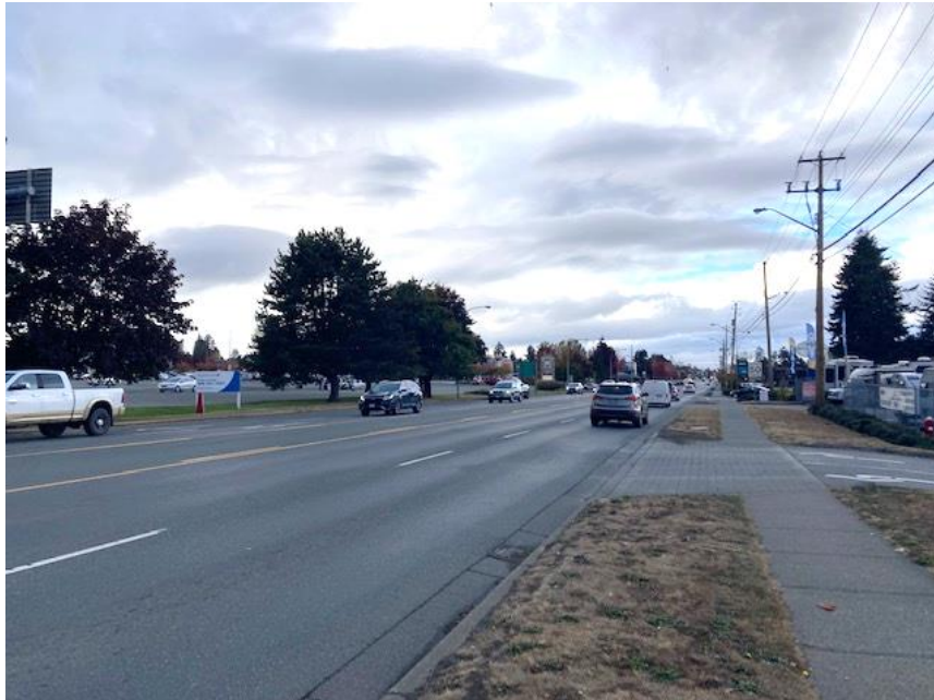
Photo 2. Proposed forcemain alignment, view looking north on Highway 19A/Cliffe Ave. in the City of Courtenay.
