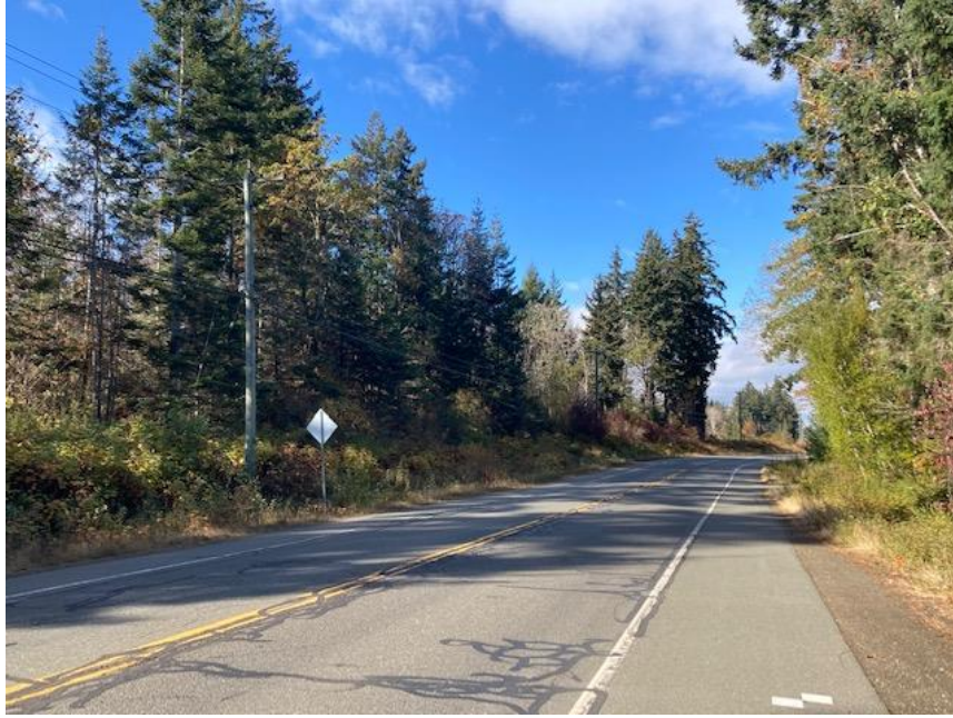
Photo 1. Proposed forcemain alignment, view looking north on Highway 19A in the Royston area.
