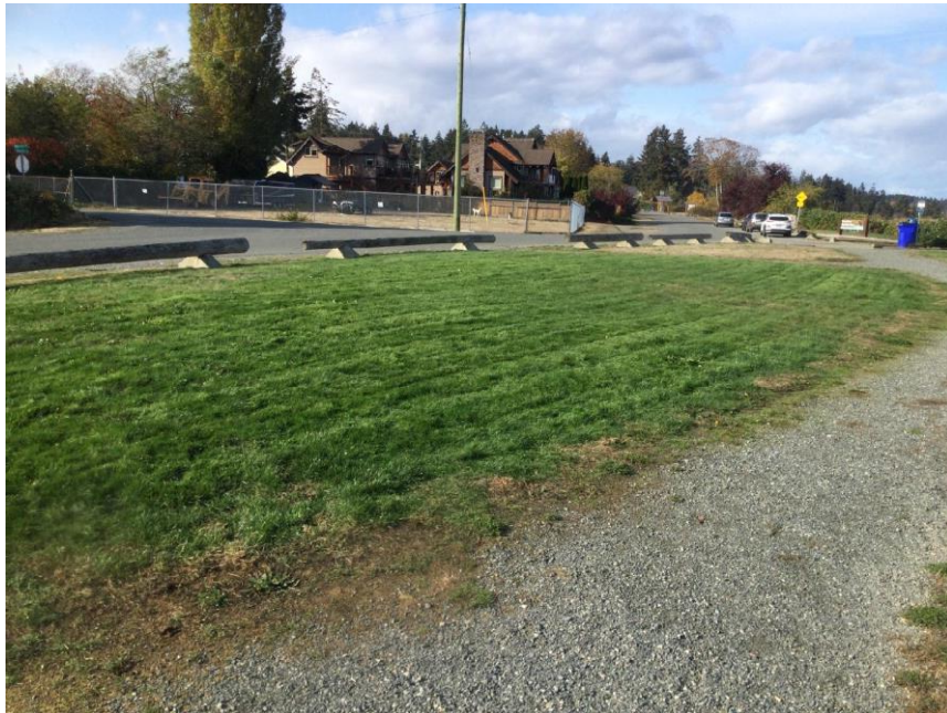
Photo 4. Proposed Pump Station 1 locations, second option located in foreground and preferred option located in back right of photo adjacent to parked cars. Fenced parcel in background was identified as a high-risk APEC with potential for contaminant migration to neighbouring sites. Records 10, 12-14 in Appendix A.
