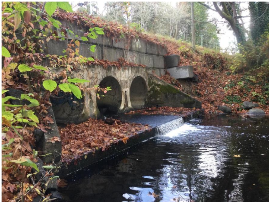
Photo 6. Millard Creek, on the downstream end of the Highway19A crossing.
